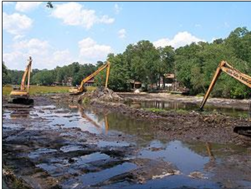
Photograph 21: Organic soils being excavated from a project site.
