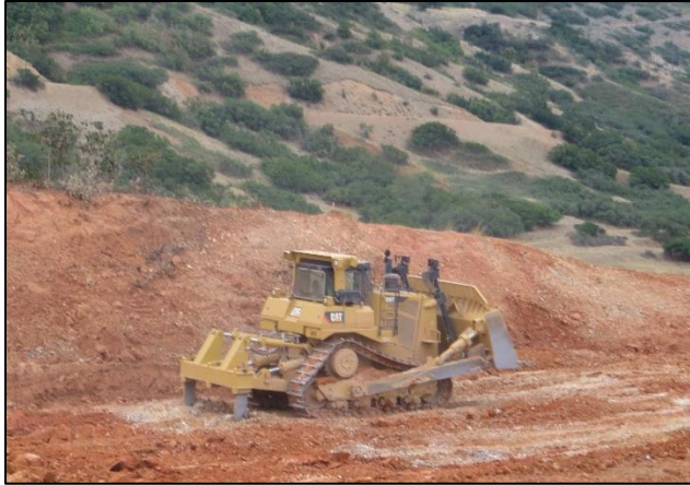
Photographs 4 and 5: Dozer with ripper attachment being used to loosen material in a cut section. Excavator with hydraulic hammer being used to remove competent bedrock from a cut section.
