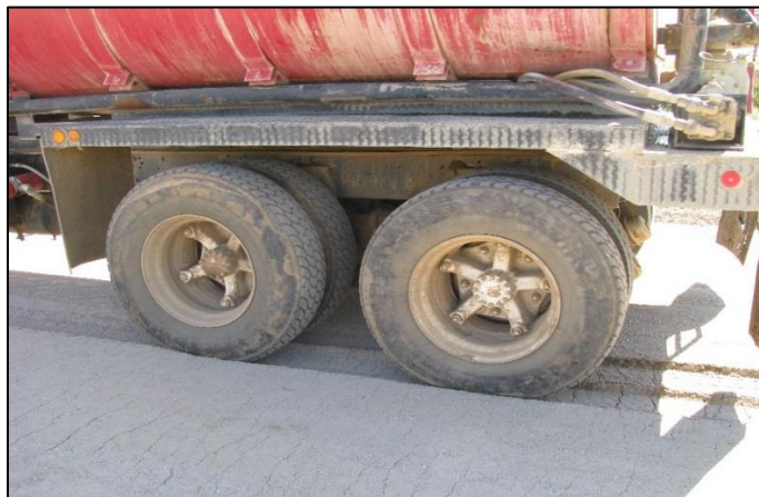
Photograph 10: Proof rolling operation being completed by a filled water truck.
