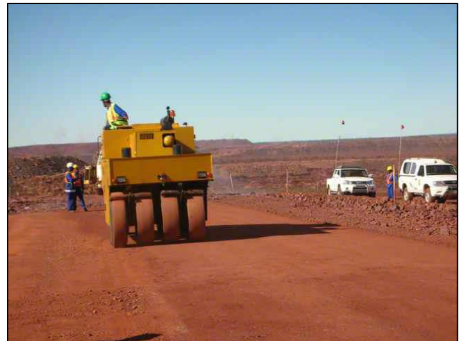
Photographs 7 and 8: Dual drummed steel vibratory roller and rubber-tired pneumatic roller.
