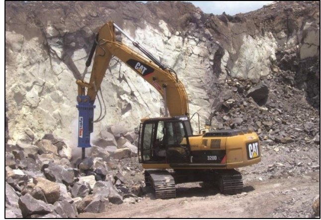
Photographs 4 and 5: Dozer with ripper attachment being used to loosen material in a cut section. Excavator with hydraulic hammer being used to remove competent bedrock from a cut section.
