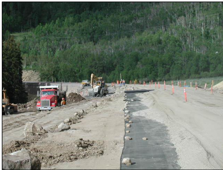
Photograph 22: Geotextile installation over soft, unstable subgrade soils.
